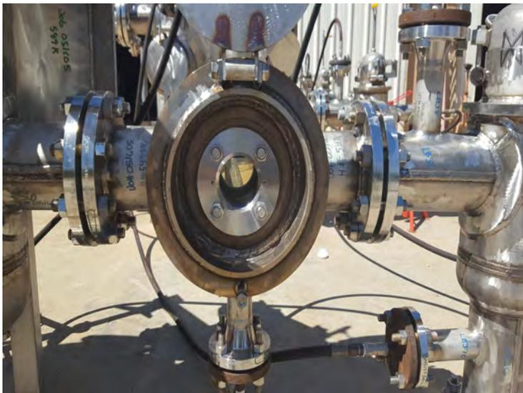
The device can be bolted on horizontally, either on the body of the Sultrap™ or flange, or vertically on the inlet valve.
